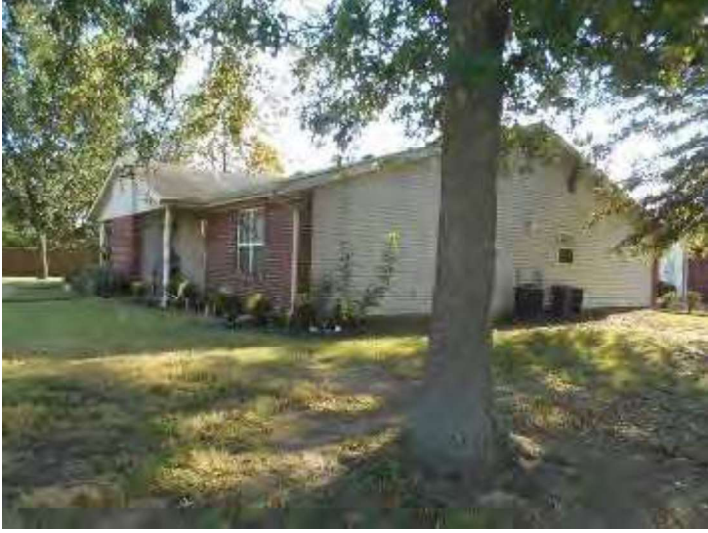
Typical Residential Building
