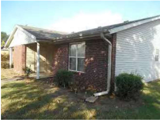
Typical Residential Building
